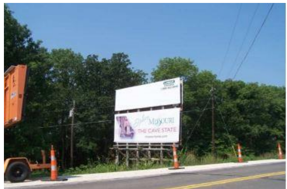
WOOD DOUBLE FACE (STACKED DISPLAYS)
