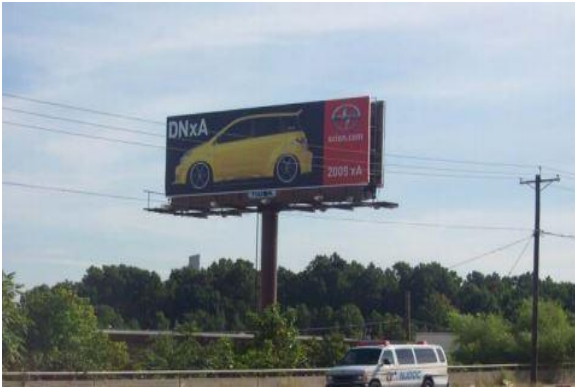
MONOPOLE DOUBLE FACE (CENTER MOUNT)
