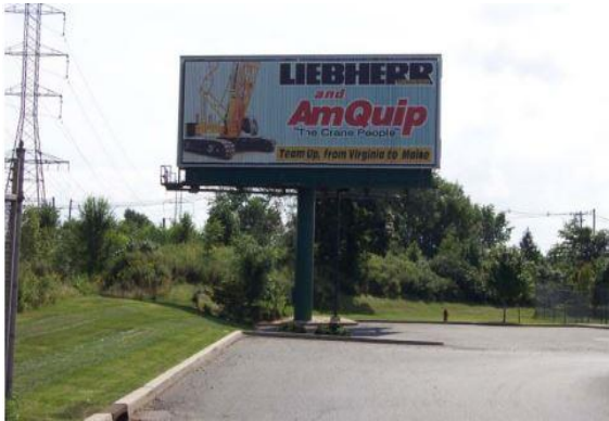
MONOPOLE SINGLE FACE (CENTER MOUNT)
