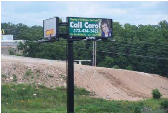
MONOPOLE DOUBLE FACE (PARTIAL FLAG MOUNT)
