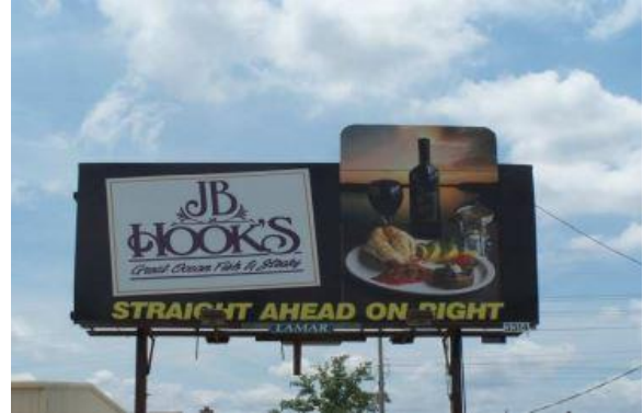
STEEL MULTI-MAST SINGLE FACE
