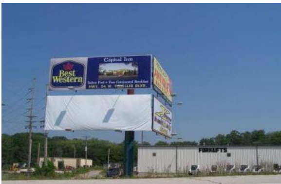
MONOPOLE DOUBLE FACE (STAKED DISPLAYS ~ PARTIAL FLAG MOUNT)
